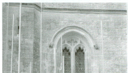
TOWER, N ELEVATION-RINGING CHAMBER WINDOW, RESTORED JULY 99.
