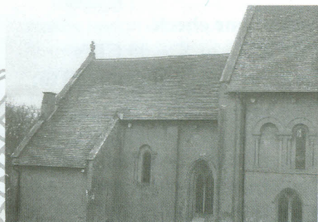
ROOF OVER CHANCEL & VESTRY. N. ELEVATION. NEW ROOF JULY 99. NOTE: Best of old tiles reused to retain character of roof.
