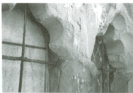
TOWER, N ELEVATION-RINGING CHAMBER WINDOW. AUGUST 98.
